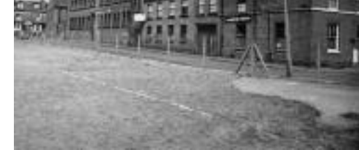
Factory buildings, looking north on Wesley St. © Image courtesy of Reg Baker and www.picturethepast.org.uk
